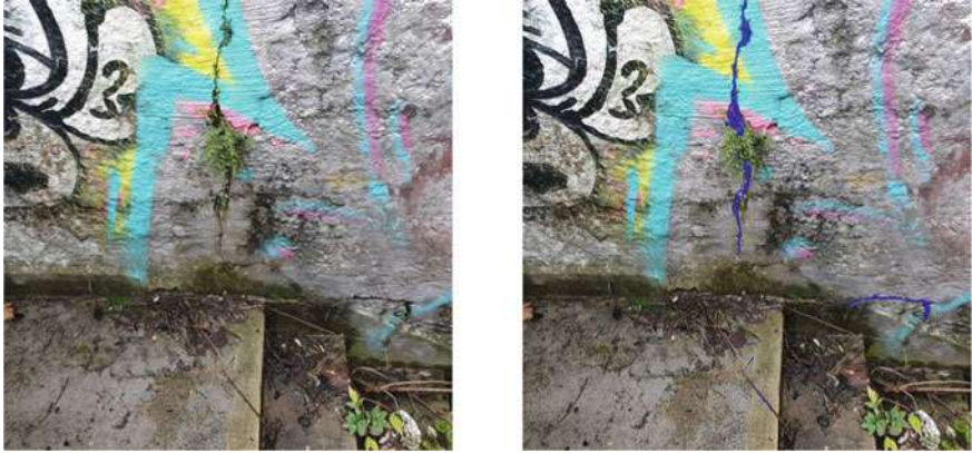
Fig. 9 Segmentation results with the FPN-Effb0 model. Blue color masks are crack predictions.
