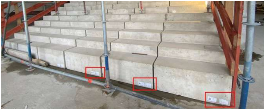
Fig. 3 Example of QR codes attached to prefabricated staircase on a construction site
