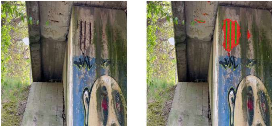
Fig. 7 Segmentation results with the FPN-Effb0 model. Red color masks are spalling predictions and green color masks are corrosion predictions.
