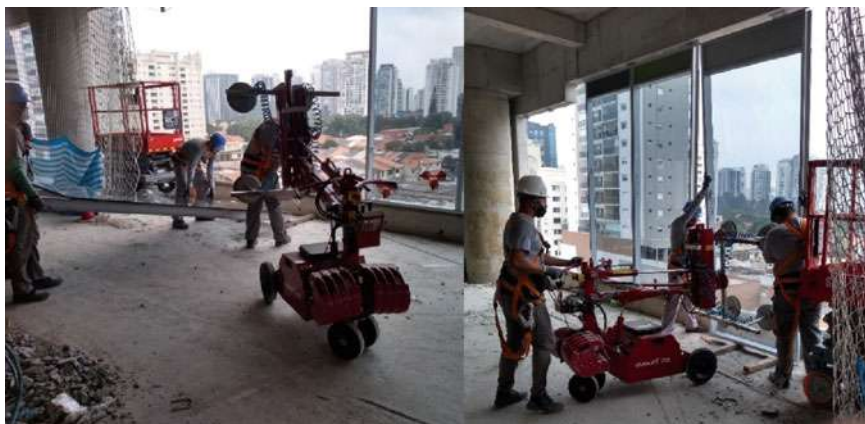
Fig. 10 Transporting and installing frame
