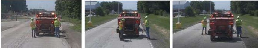
Fig. 2 Three activity classes identified for this study, crack sealing (left), transferring materials (middle), and walking (right)
