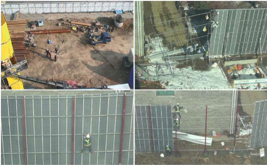
Fig. 4 Construction site scenes of the YUD-COSAv2
